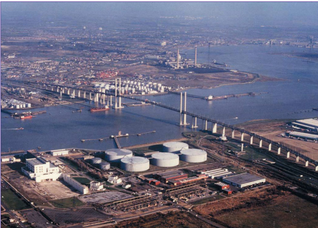
Dartford Road Bridge over the River Thames © NMR
